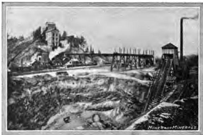
FIG. 1—CORNWALL ORE MINES No. 1 Steam Hoist to right; Robersonia Hoist in center near tracks; No. 2 Hoist and substation on hill; Ore bin and Stockpile in middle.
